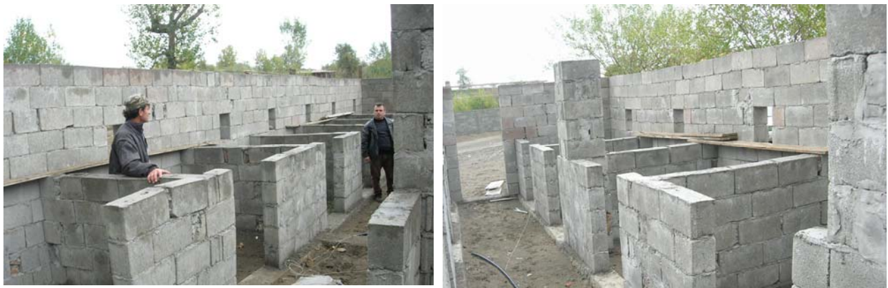
The new stable in construction process
